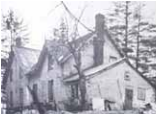
Before demolition (1945) Photo: Kitchener-Waterloo Record
